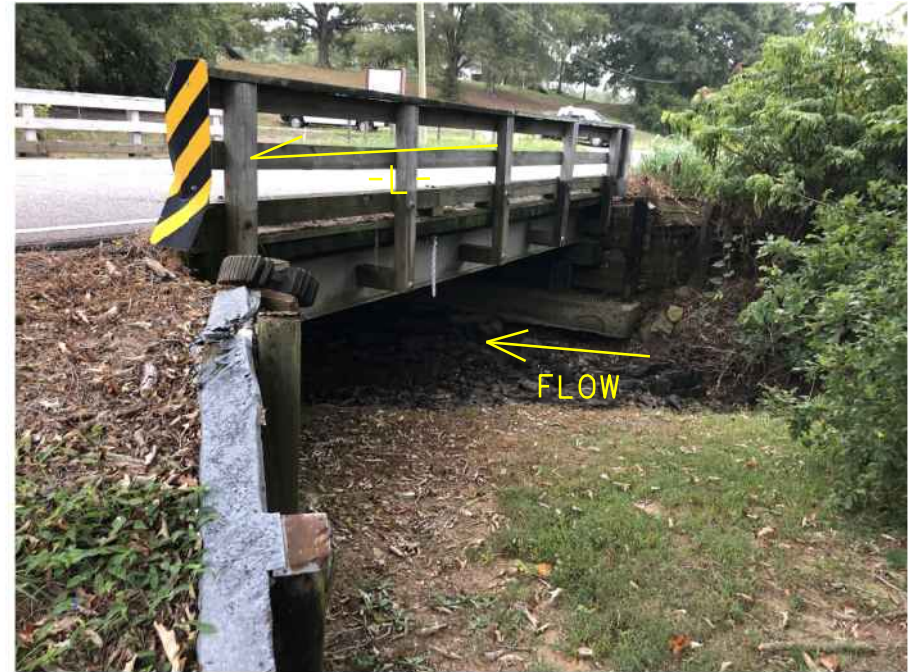
Photo #1: Bridge 093 End Bent 2 looking south (downstation) towards End Bent 1
