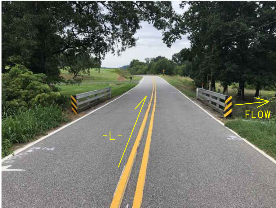
Photo #1: Bridge 093 End Bent 1 looking north(upstation) towards End Bent 2
